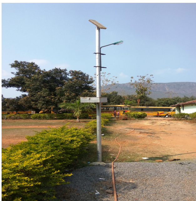
Solar Street lightning using MPPT algorithm
